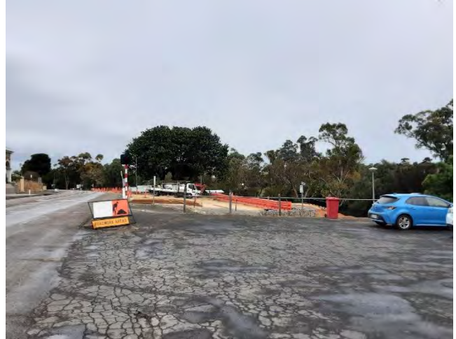
Photo 18 View from Burra Town Hall facing north
