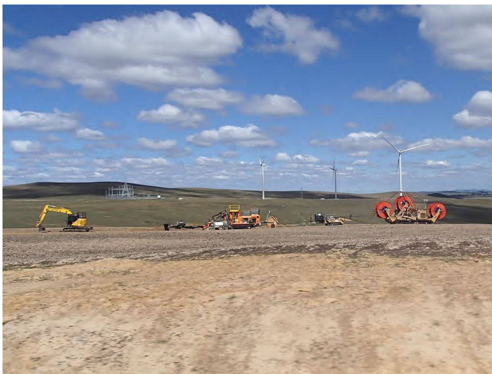
Plate 7 Cable laying equipment (Image: ©GBD 2023)
