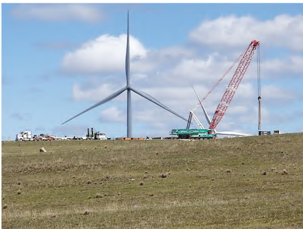
Plate 8 Typical crane plant utilised in wind turbine construction (Image: ©GBD 2023)
