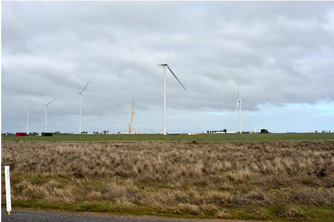
Plate 5 – Typical wind farm under construction (Image: ©GBD 2017)
