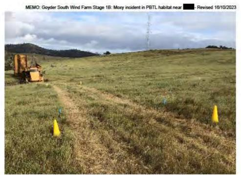
Figure 3. Micro-sited corridor, marked with blue marker pins and orange marker paint.
