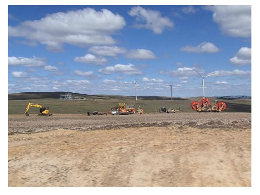
Plate 7 Cable laying equipment (Image: ©GBD 2023)
