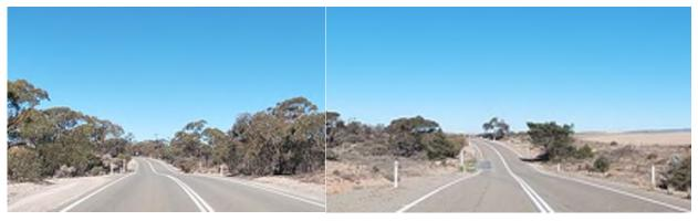
Figure 3-8: Vertical geometry constraints looking south along the Worlds End Highway. Constraint 1 located south of Hallelujah Hills Road (left), constraint 2 located north of Powerline Road (right).
