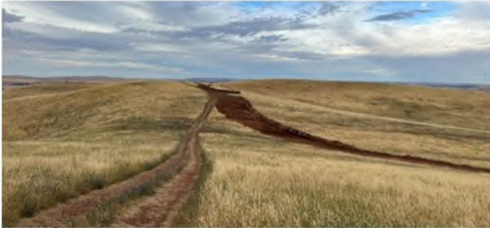
Figure 3. General photo looking [REDACTED] showing alignment that was cleared.
