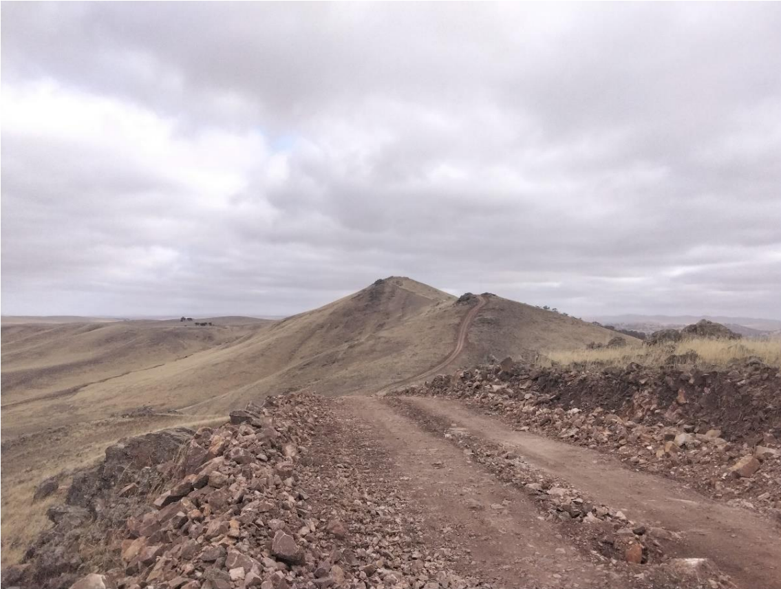
Figure 2-7 Typical site conditions along the proposed WTG corridors (site SG025, looking south)
